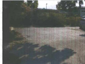
Area 6 – Excessive Pavement
